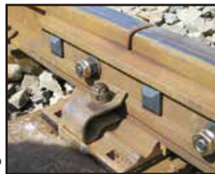
Installed with HARDLOCK nuts
